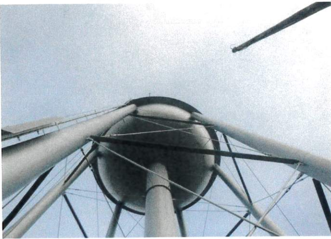
Exterior Coating Under Belly
