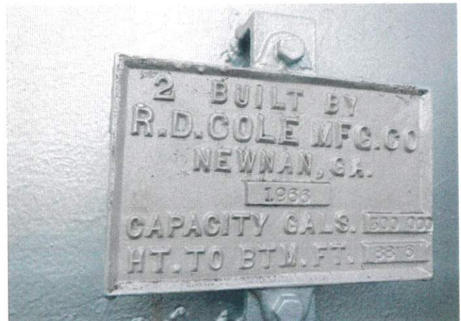
Tank Identification Plate
