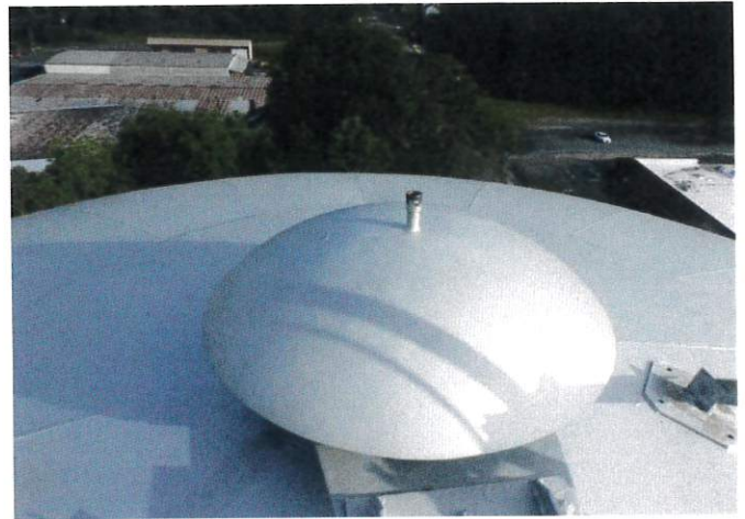
Exterior Coating Roof
