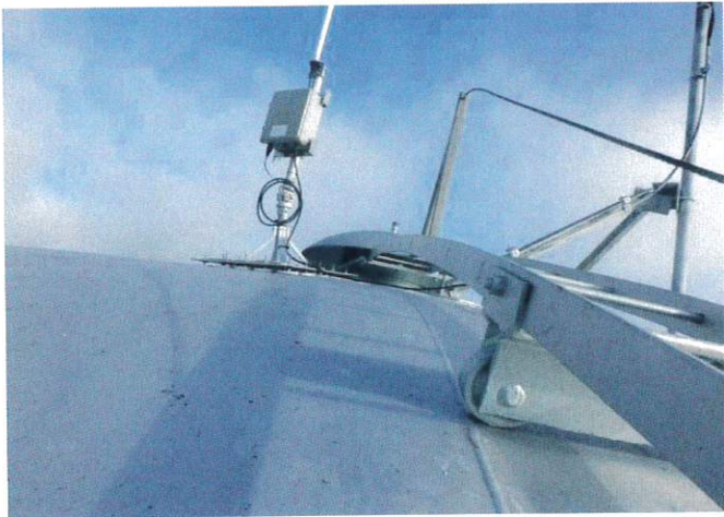
Exterior Coating Roof
