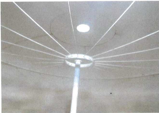
Interior Roof Structure
