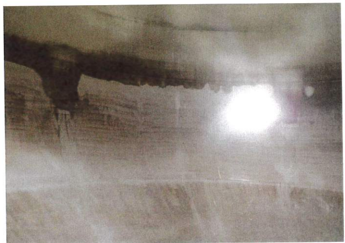
Interior Coating Sidewall
