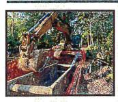
The Phase 2 rehabilitation is a continuation of the efforts completed by Phase 1. Phase 2 consists of digging and replacing approximately 7,000 feet of 24" gravity sewer, and approximately 1,500 feet of 24" cured-
