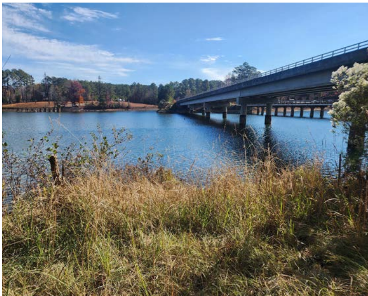
North side of Lilly’s Bridge
